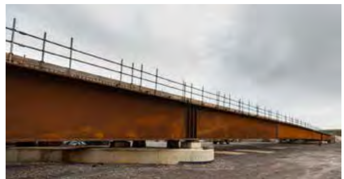
Nash Lee Road Overbridge girders, November 2025 4
