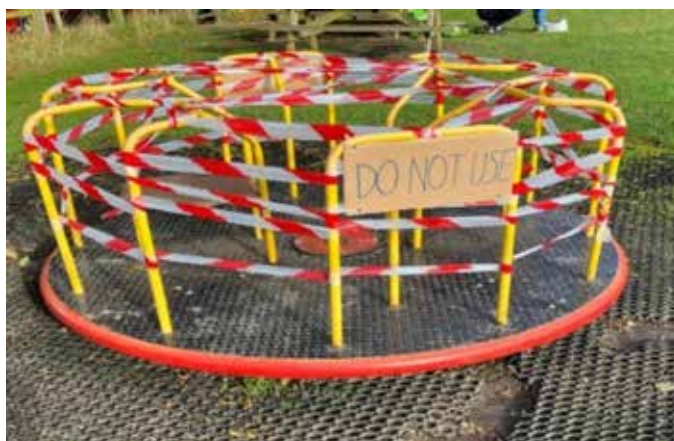
Roundabout condemned as potentially a head injury risk as matting underneath was worn out.
